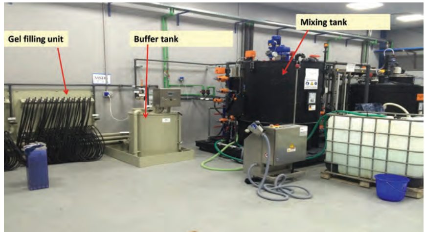
Gel Mixing and Circulation System – Actual Installation
