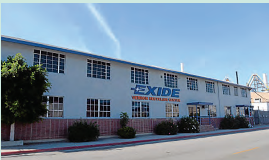
Exide Technologies' recycling plant in Vernon, California closed in 2013
